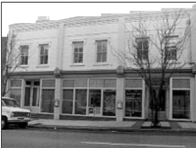
The storefront bays with their decorative mid-cornices and bands of glazed transom panels contribute to the architectural character of this Hargett Street commercial building.
