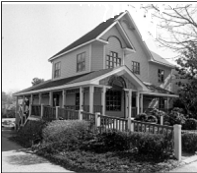
Both the use of traditional materials and details and the addition of landscape screening successfully integrate this ramp with the building and its site.
