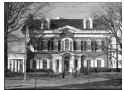
GEORGIAN REVIVAL STYLE Capital Area Visitor Center Andrews-London House, 301 North Blount Street
