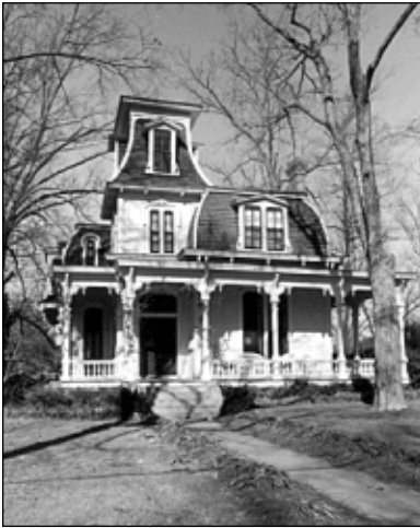
SECOND EMPIRE STYLE Heck-Wynne House, 511 East Jones Street
