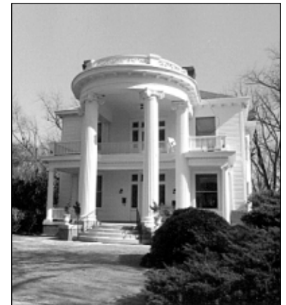
NEOCLASSICAL REVIVAL STYLE Tucker House, 418 North Person Street
