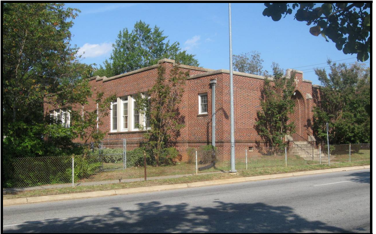
West and South facade
